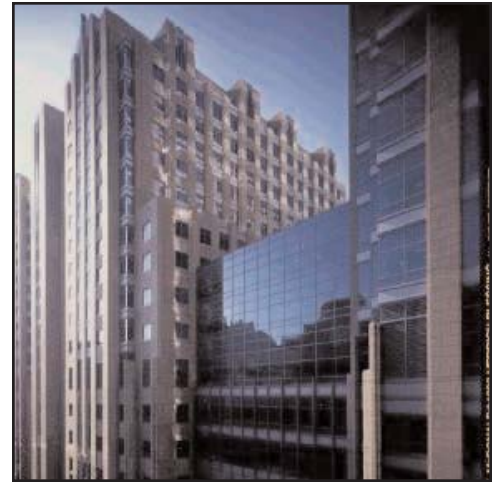
Northwestern Memorial Hospital
